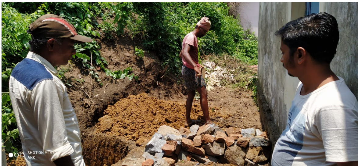
Figure 3: Construction of Toilets in Quarantine Center of Tankachhai GP (Purusottampur block)
