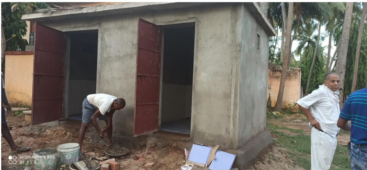
Figure 7: Construction of Toilets at Kanheipur Gram Panchayat (Khallikote Block)
