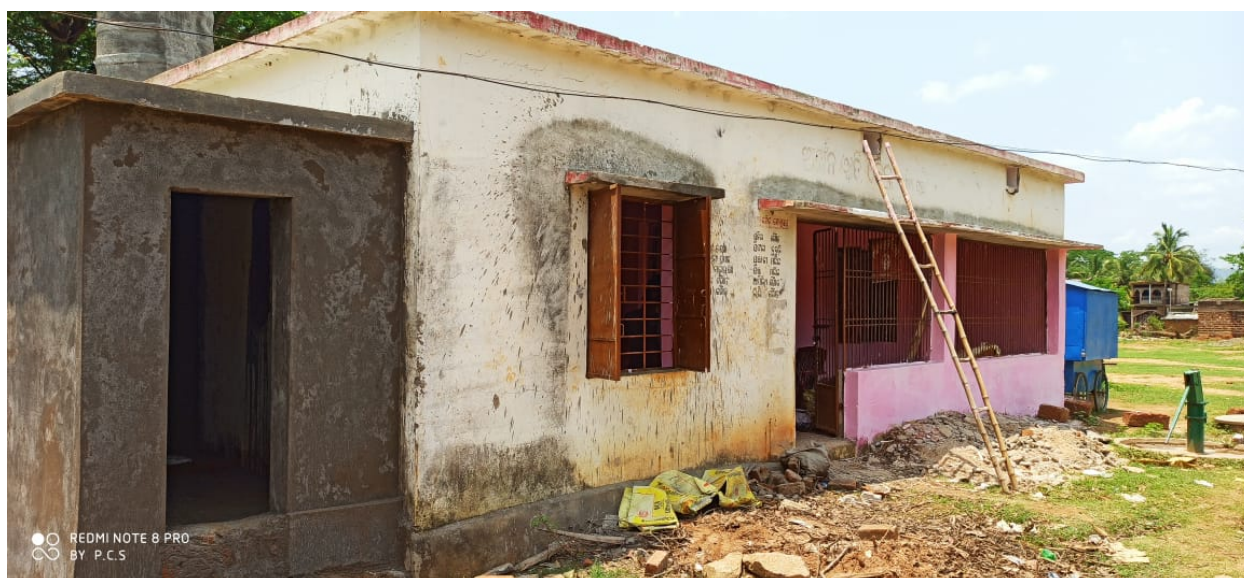
Figure 2: Refurbishment of Quarantine Center at Manikyapur GP, Khallikote Block
